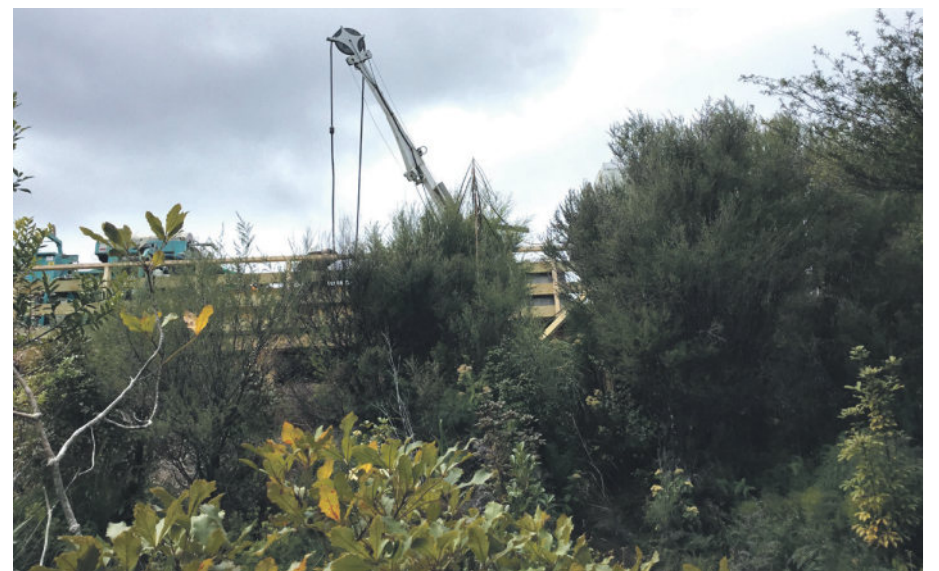
The latest drilling site set up above the waterfall, Parakiwai valley.
